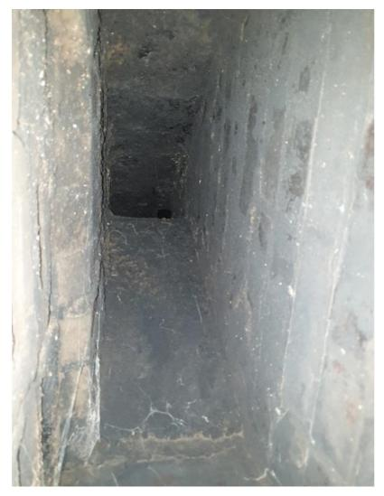
The chimney starts at the top of the firebox and extends vertically through the roof of the house. The chimney must protrude a certain distance above the roofline of the house to ensure sufficient draw on the fireplace.
