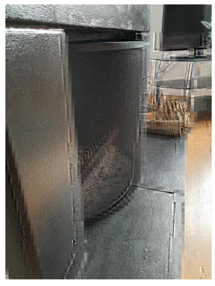
As a hearth has to deal with high temperatures, it so also needs to be made from non-combustible materials. Common materials used as a hearth include granite, marble, stone, concrete, brick, ceramic and quarry tiles.
