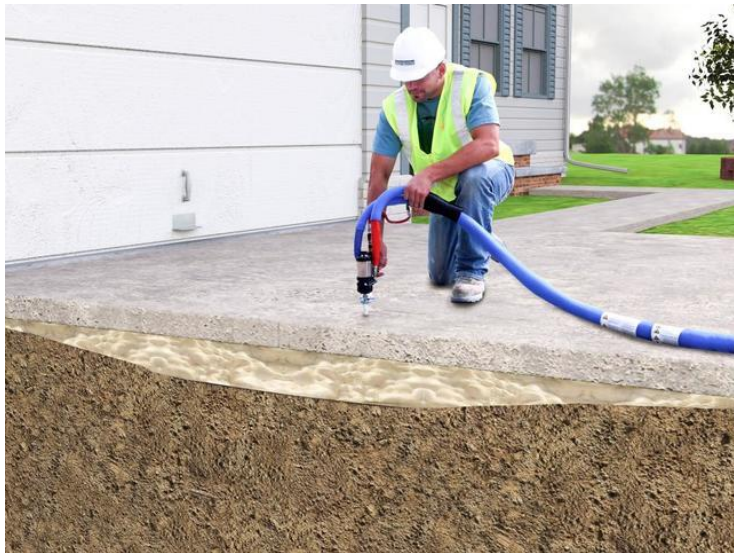
Installer injecting polyfoam
